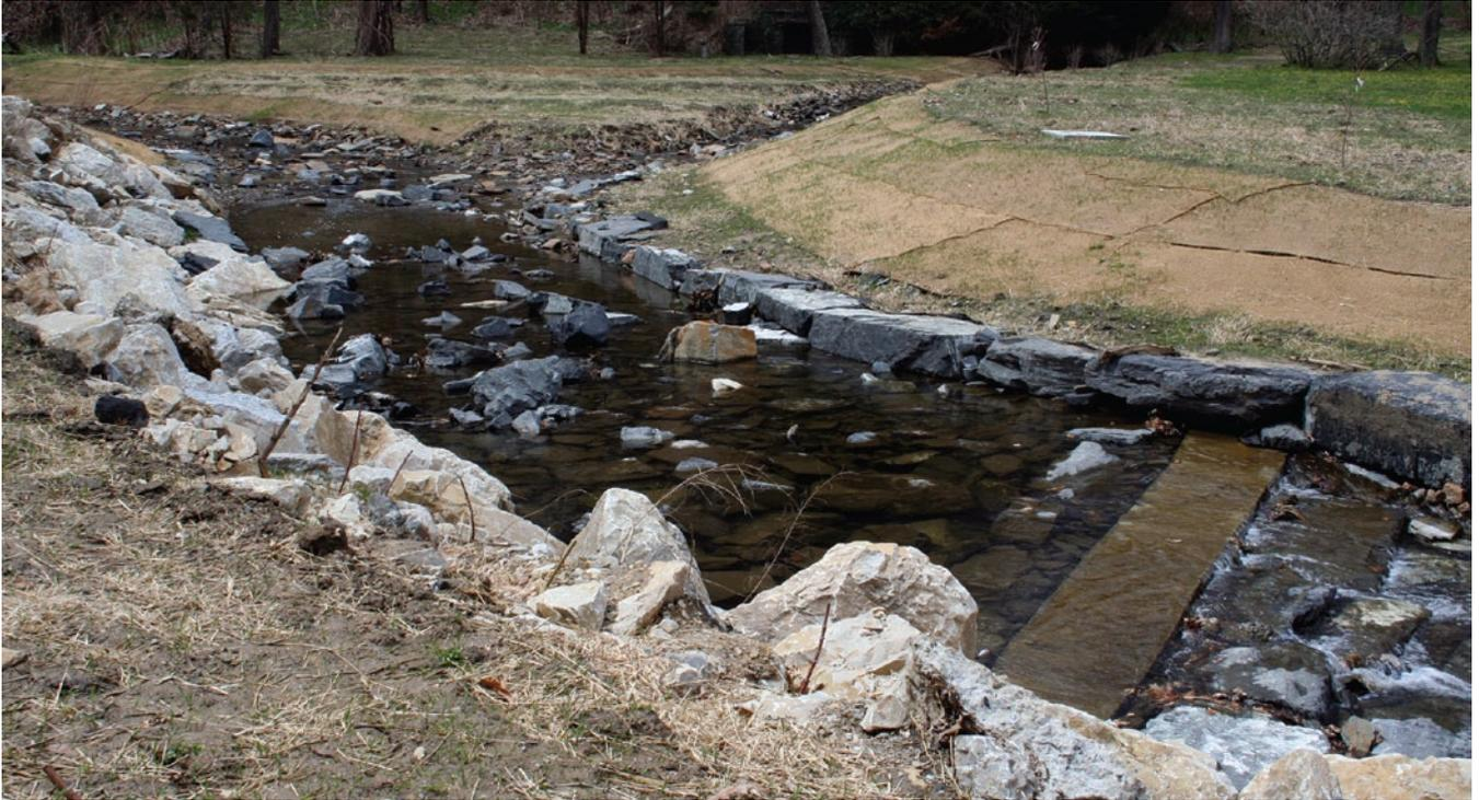
**A residential work in progress: an attempt to re-create Mill Creek's desire for a gentler bank along its steeper side, with regrading and seeding in the floodplain. Some hardscaping remains, but damage will be less severe with reduced restriction of the creek's flow.**
