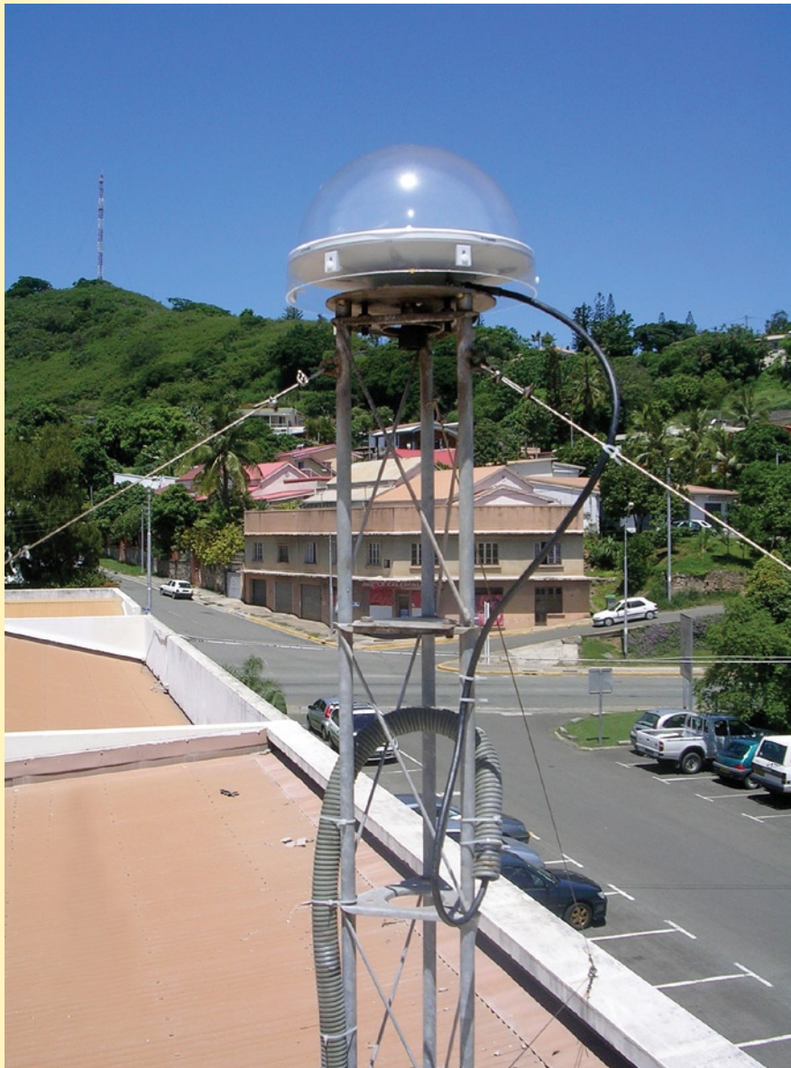
Located in Vallée du Tir (Nouméa), a permanent Trimble NetRS/ZGA with weather radome is part of the future BGN Trimble VRS infrastructure network.
