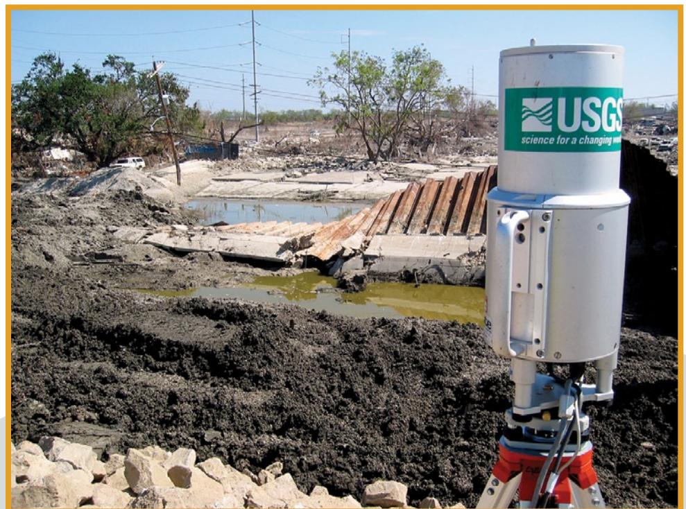
LIDAR unit at Lower 9th Ward, northern levee breach on the Inner Harbor Navigation Canal. Photo: Robert Kayen
